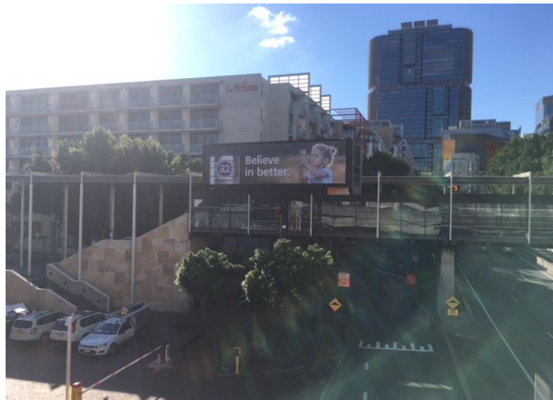
south side of existing billboard
